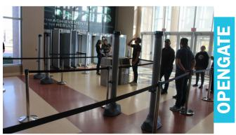
OVG 360 upgraded the Alerus Center security magnetometers to the CEIA Opengate system which drastically improves traffic flow into the venue for busy events.
